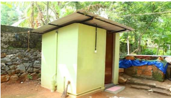
Construction of Toilet
